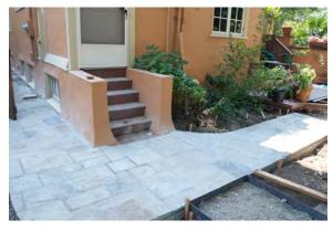
A concrete slab is poured to top with mortar-set stone, which will "breakaway" into sand set stone.
